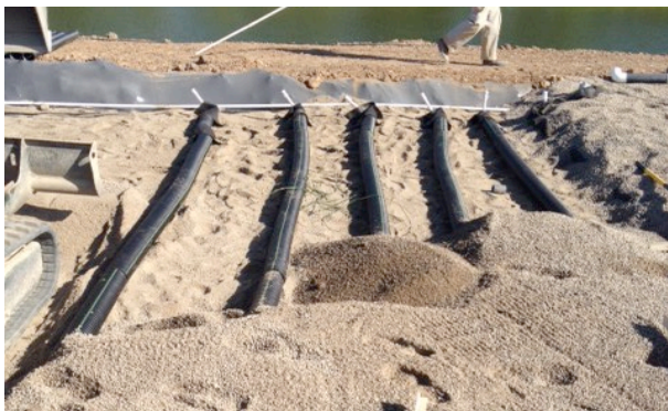
Figure 2: Filled cell with distribution piping
