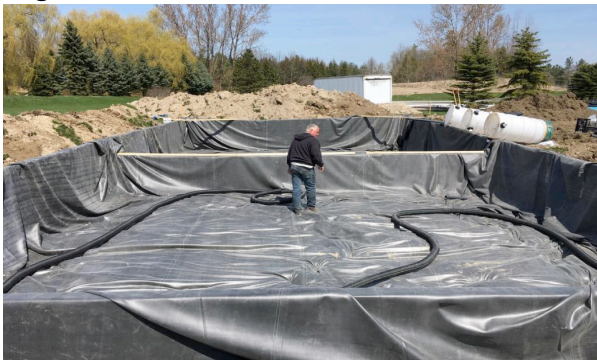
Figure 1: Cells with impermeable liners and collection piping
